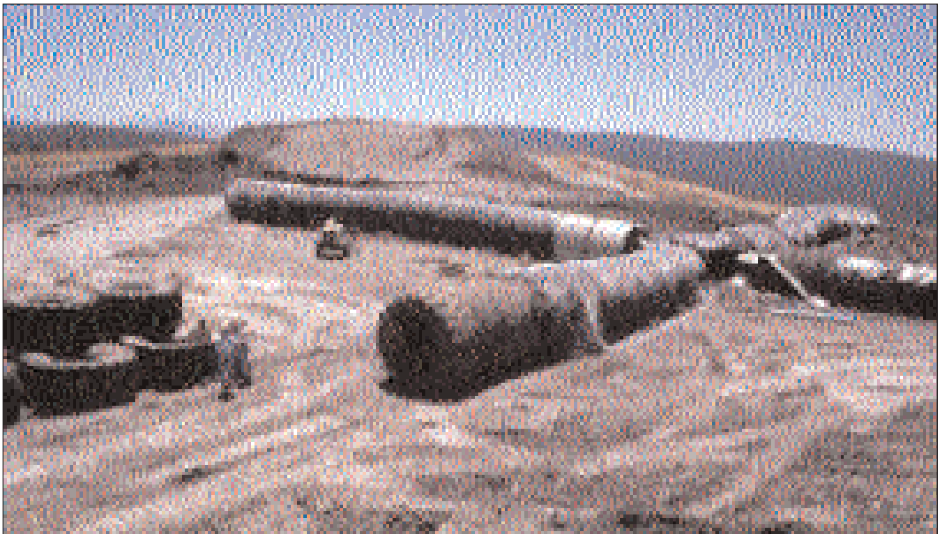
At Homestake Mining Company’s McLaughlin Mine in California, surplus truck tires were buried beneath waste rock to create an innovative and cost-effective bat roost. If careful consideration is given to design and construction, artificial structures can provide important roosts for bats.
